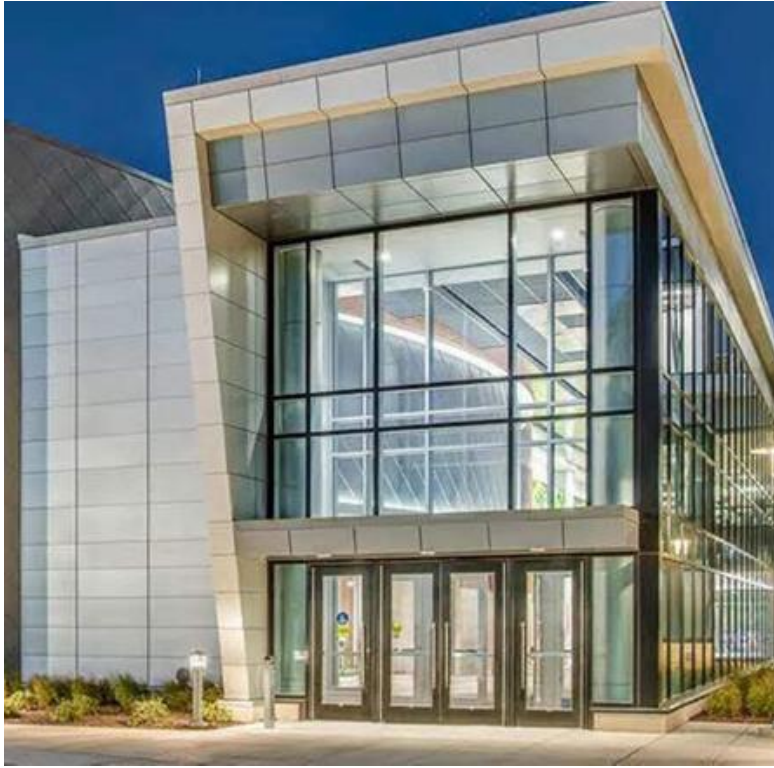
The Audion: Tower at STAR Campus
